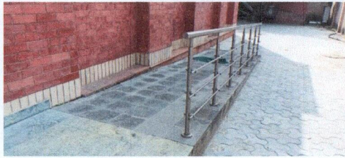
Image 13: Ramps with one sided handrail was observed at the entrance of the buildings.
