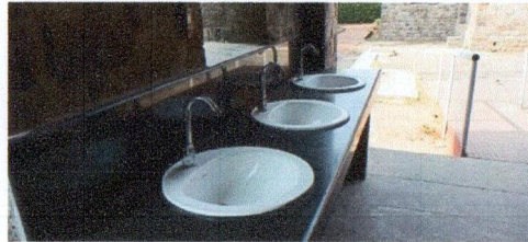
Image 10: Lavatory faucets observed on site without aerators.
