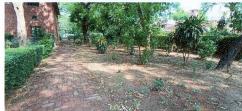
Image 3: Brick paving was used on Pedestrian walkway
